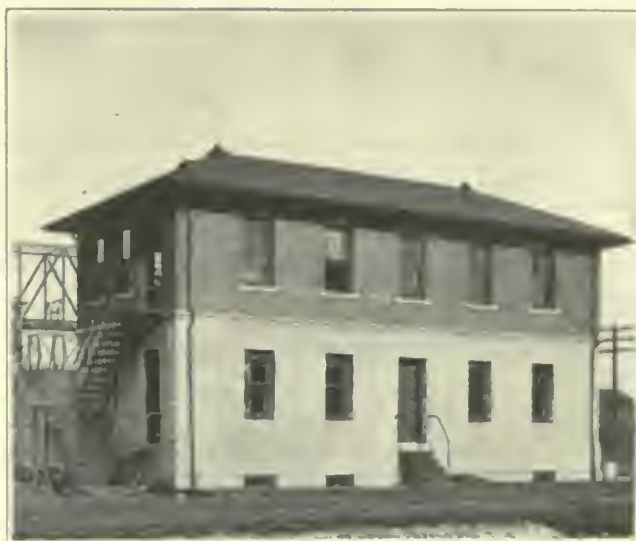
FIG. 293. INTERLOCKING PLANTS. Interlocking tower of the Lake Shore & Michigan Southern Railway west of Indiana Harbor Station. This plant controls signals governing the lift bridges over the ship canal.
